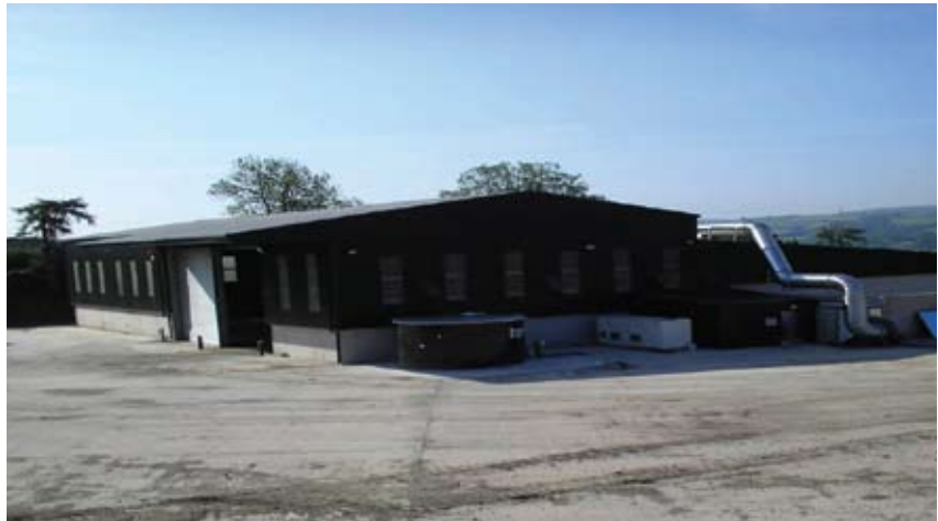
Funding provided in Wales means this £1.3m in-vessel composting facility is one of three regional demonstration facilities being developed
